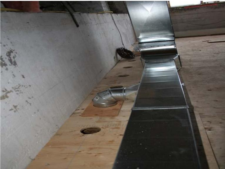
Air Gap Supply and Return Ducting
