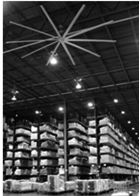
Figure 14. Large HVLS circulating fans in a warehouse
