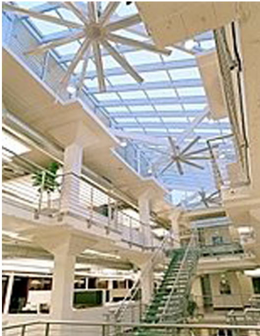
Figure 15. Atria with circulating fans for destratification
